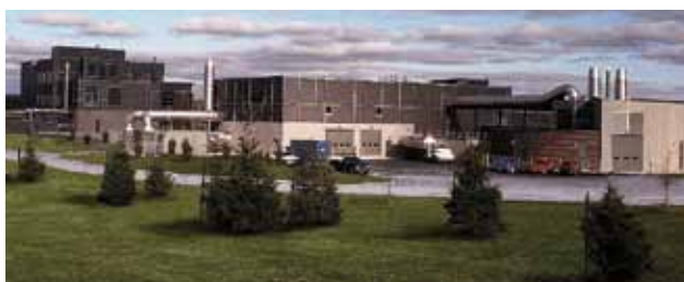
The organic waste conversion facility will be built on the site of the La Pinière water treatment plant.
