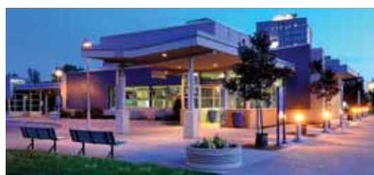
Design for the waiting areas at the Le Carrefour bus terminal in Laval
