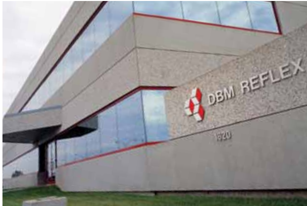
Head office of DBM Reflex Enterprises and DBM Reflex Lighting Solutions in Laval.
